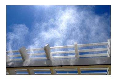
Misting Stations spray a fine mist of water into the air. Misting stations are an effective method for preventing heat-related problems. As the water evaporates, it absorbs heat from the surrounding air, thereby lowering the overall temperature of the air. Misting stations can be effective in large areas such as athletic fields and playgrounds.
