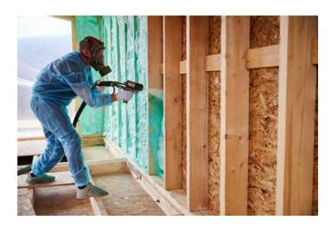
Improve Building Envelope by focusing on air-sealing, utilizing high-performance insulation materials, and minimizing thermal bridging. Thermal bridging occurs when structural elements like studs conduct heat through insulation. Thermal breaks are materials that interrupt the flow of heat; which can be accomplished by placing insulation on the exterior of the framing.
